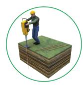
Self connectable rods: The lower end of each rod is equipped with a point used both for driving into the earth and for connection; the upper pierced end receives (without the sleeve) the point of the previous rod. Use a rivetting head so as not to damage the upper end when driving in.
