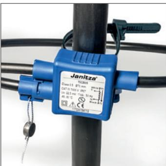
Sealed and mounted on the phase conductor with a cable tie
