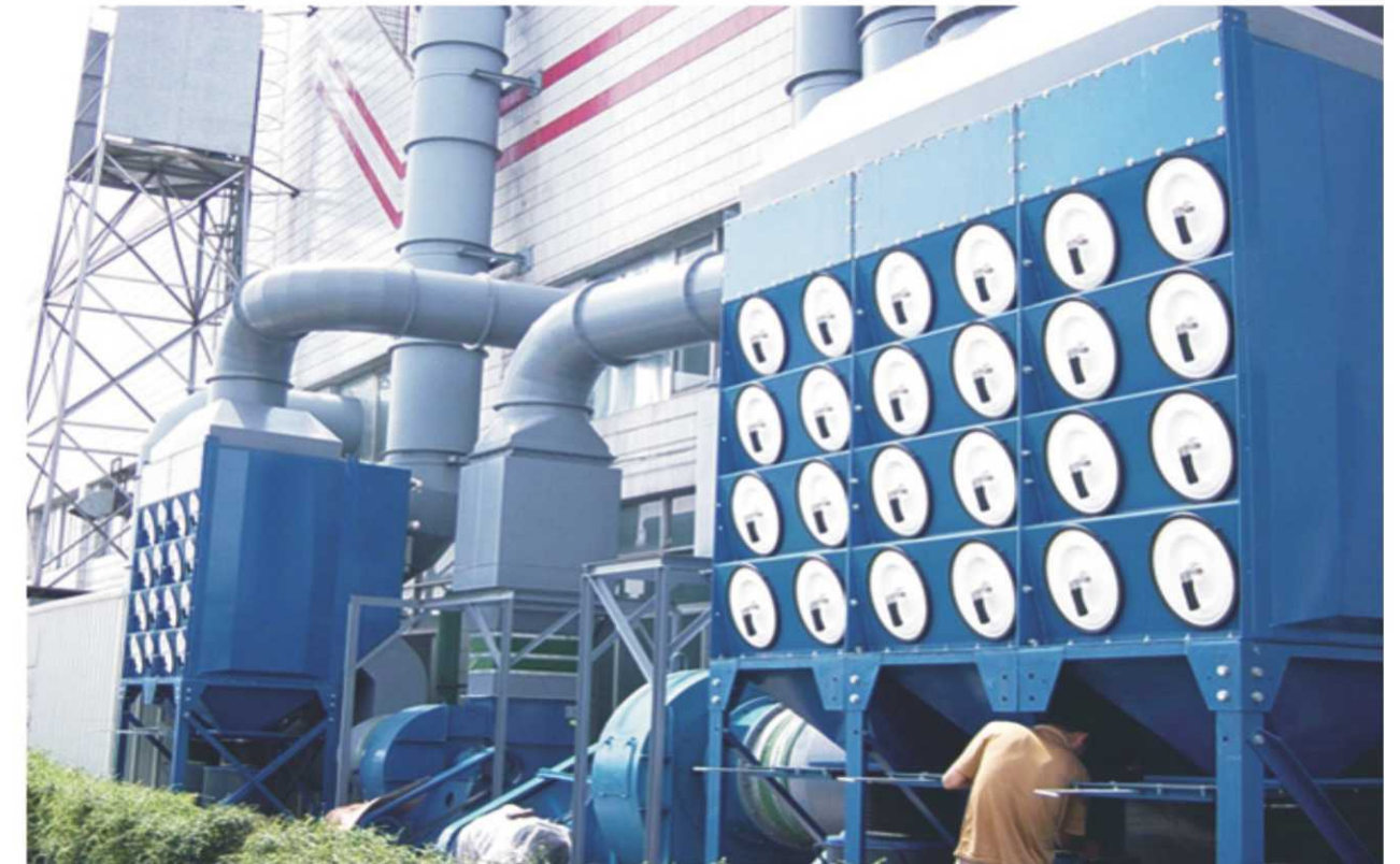
▲ Welding Fume Filter Cartridge Centralized Dust Removal System for Automobile Manufacturing Plant
