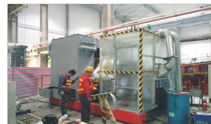
Installation and Commissioning of Mobile Polishing Room Dust Collector
