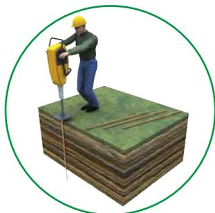
**Self connectable rods:** The lower end of each rod is equipped with a point used both for driving into the earth and for connection; the upper pierced end receives (without the sleeve) the point of the previous rod. Use a rivetting head so as not to damage the upper end when driving in.
